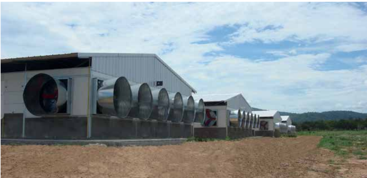
Tunnel ventilation (fan with cone)
