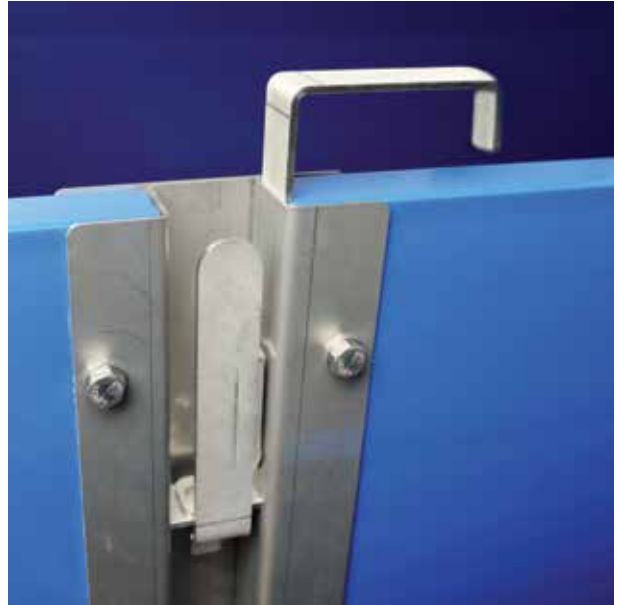
One-handed lock of gate at the piglet pen
