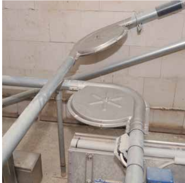
Deflecting corner made of stainless steel
