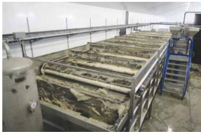
Flotation tanks
