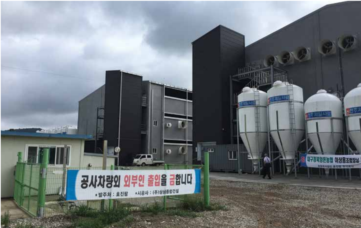
At the Hyojin farm, 17,100 pigs are housed in two buildings on 3 levels each. The farm features 2 freight elevators for the animals and one bridge for moving.
