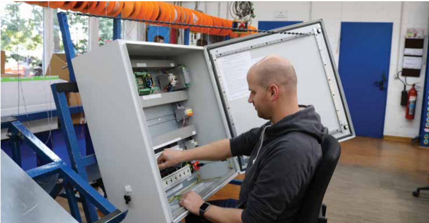
Customised switch cabinet construction
