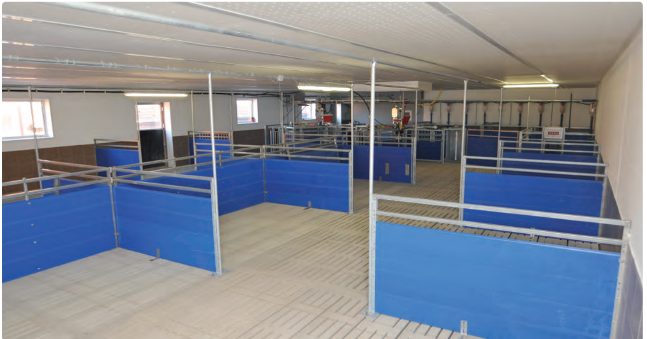
The SowComp enables individual feeding which meets with the requirements of sows in group managements.
