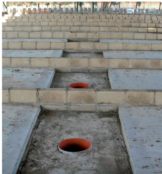
Fundament in rawness
