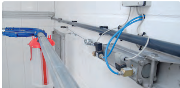
Automatic release mechanism for the volume dosificator
