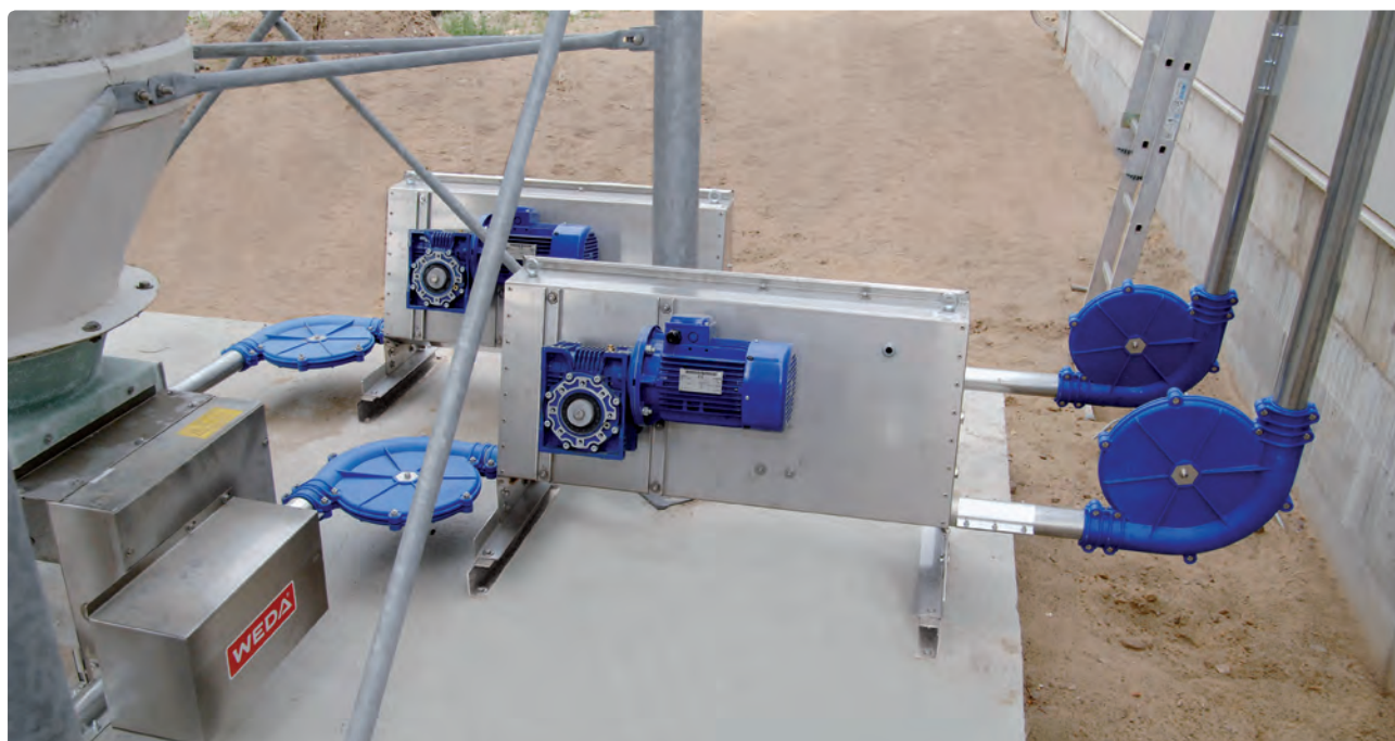
Conveying of dry components outside the house
