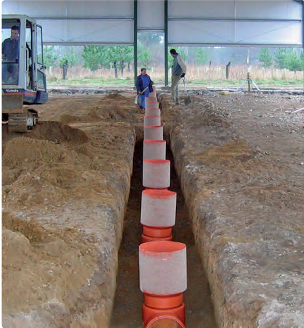
Excavation of the liquid manure channel and alignment of the pipes
