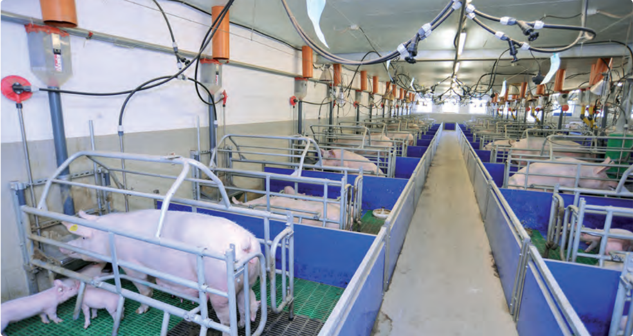
Fresh Nose Ventilation
