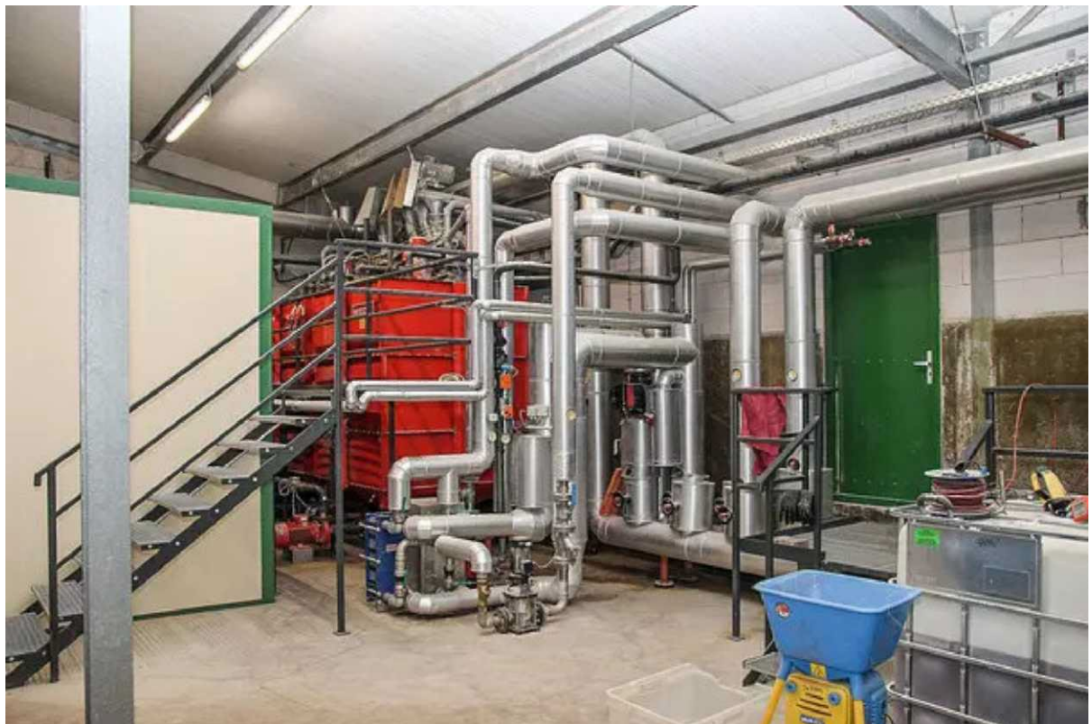
All components are mixed in the premixing tank before the ferment mixture is pumped over. (Image source: Asten)
